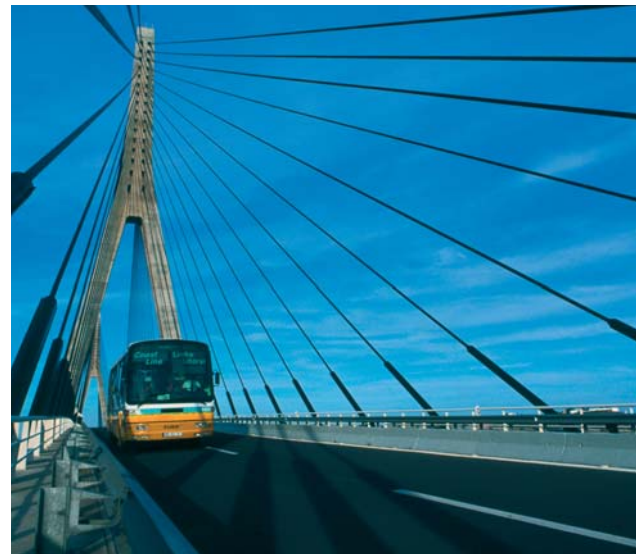
Bridge linking Spain and Portugal over the Guadiana river, Algarve, Portugal.
